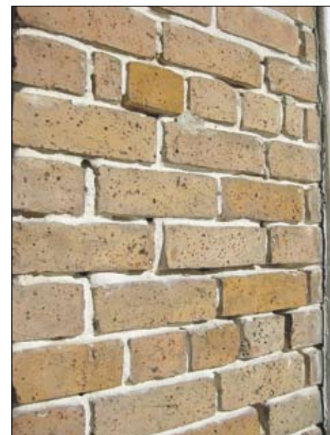
If your mortar looks like this: a powdery, sandy white substance, do not be alarmed. The mortar has simply reached the end of its life cycle. Hire a mason knowledgeable about historic brick, and he can restore your masonry structure in a process known as repointing.
