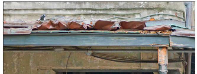
The edge of the roofing at this gallery is bent and not secure. Strong storm winds can peel the roof off of the building.
