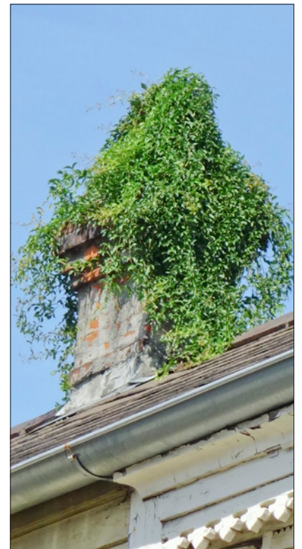
The vines on the chimney can clog the flue and dislodge the mortar.
