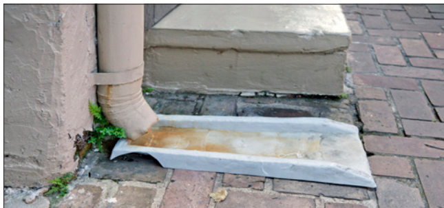
A splash block can direct storm water from a downspout away from a building.
