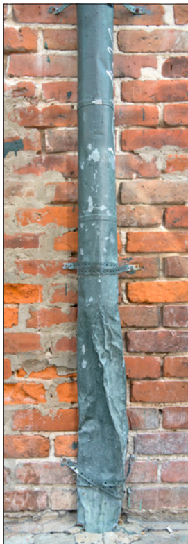
The crushed downspout is impeding water flow.
