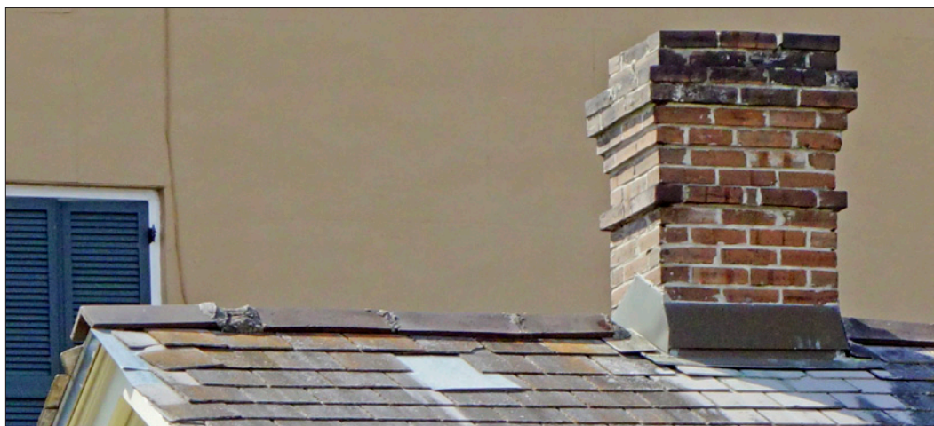
Prior roof patching evident in multiple roof locations. Note the poorly executed expanded ridge joint repair of the ridge tile.
