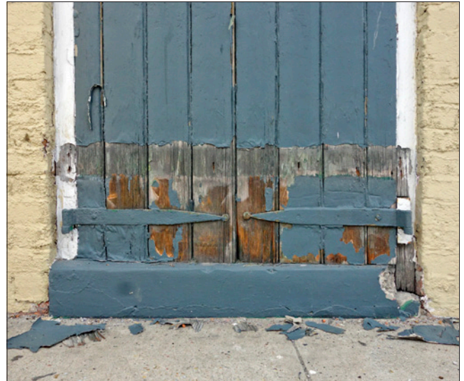
Improperly maintained paint along the bottom of the door leaves the door susceptible to damage from moisture, termites and other pests.
