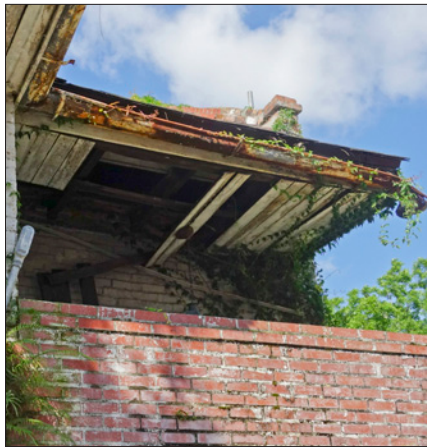
Damage is evident along the roof overhang due to moisture infiltration. The gutter has been dislodged, several soffit boards are missing or displaced, and vine growth is progressing on and between building components.
