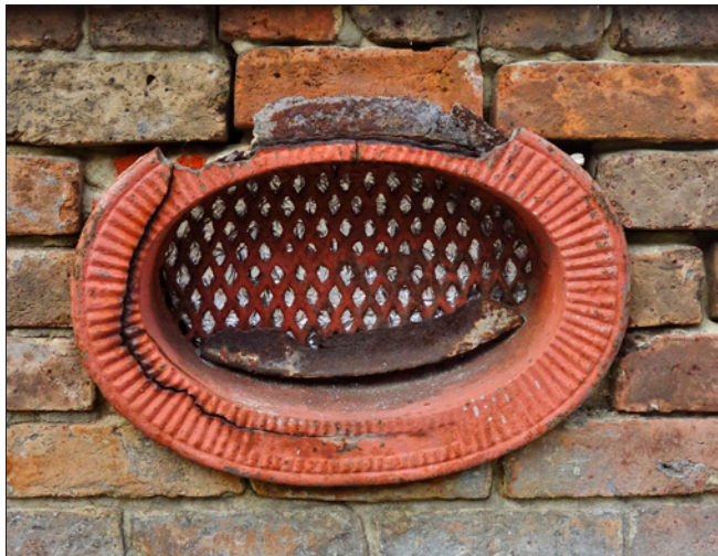
The foundation vent is cracked, rusting, and the grille has been blocked from behind reducing air circulation in the crawlspace. Also note the loss of mortar at the brick joints.
