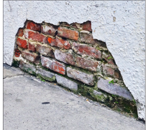
The stucco is cracked to revealing loss of mortar and brick damaged by water infiltration.
